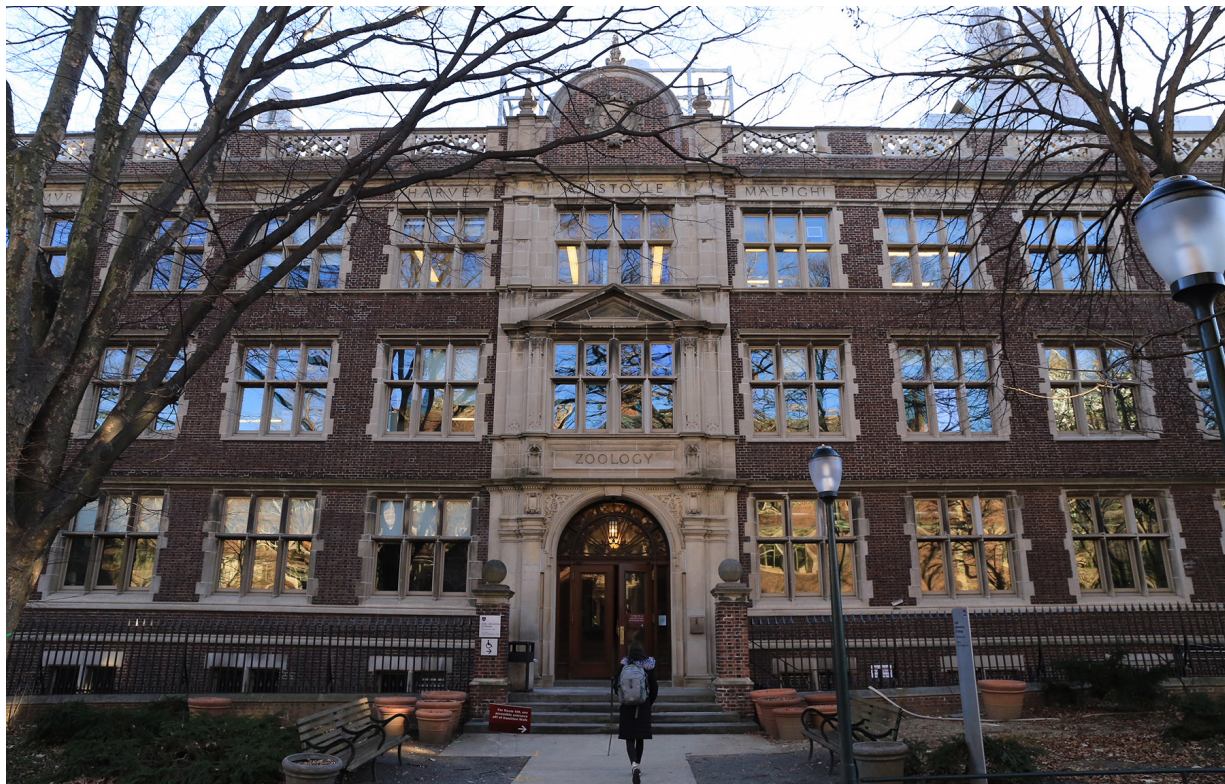
The Century Bond program has funded the replacement of Leidy Laboratory's HVAC system in an effort to improve energy efficiency.
