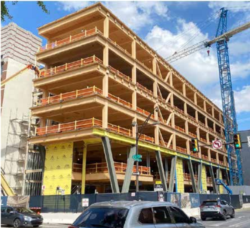
Amy Gutmann Hall, completed in 2024, is Philadelphia's tallest new mass timber building, with a cutting-edge system that significantly reduces the building's carbon footprint – by 52% relative to concrete, and 41% relative to steel.
