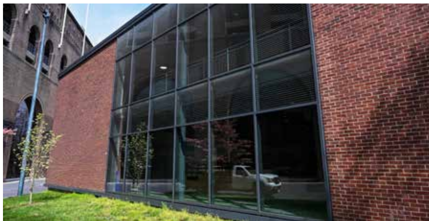
Ringe Squash Center features bird-friendly glass to reduce bird strikes as part of Penn’s bird-friendly efforts.
